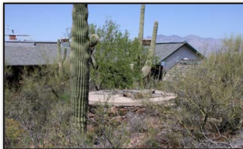
Figure 41. No longer in use, this abandoned cistern (center) held an important water source, rainwater captured from the roof of the laboratory.
