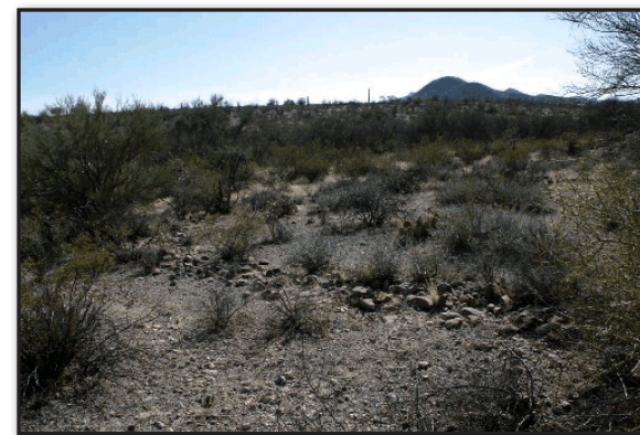
Figure 20. This rock alignment, which extends across the slope, retains soil and moisture. Check dams are similar in appearance to this, but block small drainages.
