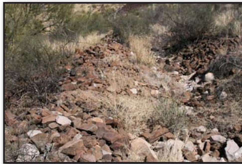
Figure 23. An early wagon road on the western slope made by removing rock down to white hardpan.
