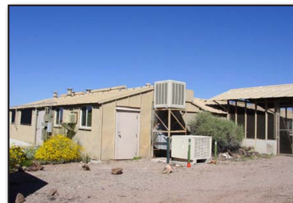
Figure 46. One of several metal structures moved to the hill after 1940.
