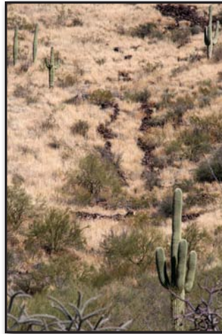
Figure 28. Rock chute (center).
