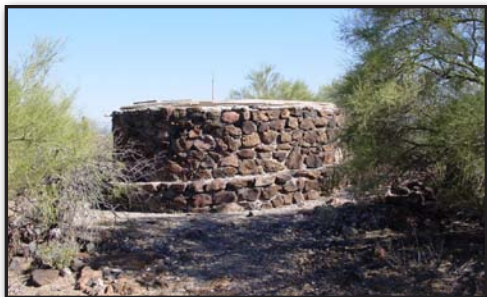
Figure 40. Constructed of local field stone and concrete, this storage tank held water pumped through several thousand feet of pipe from a well on the floodplain of the Santa Cruz River.
