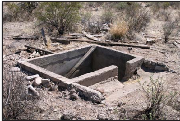
Figure 48. An elaborate concrete-lined pit that appears to be a water catchment and measuring device.
