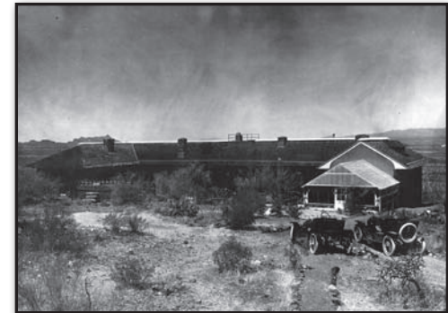
Figure 34. This picture, ca. 1911, shows the 1906 addition that made the building U shaped with a greenhouse (right side front).
