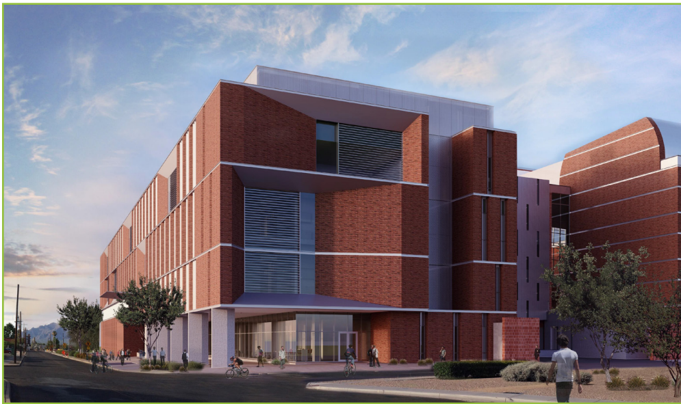
Bioscience Research Laboratories. Project is currently under construction with scheduled completion being February 2018
