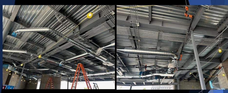
Overhead MEP is ongoing in Multipurpose Room Building. Fire sprinkler lines, ductwork & electrical conduits. Field and virtual coordination has gone smoothly.
