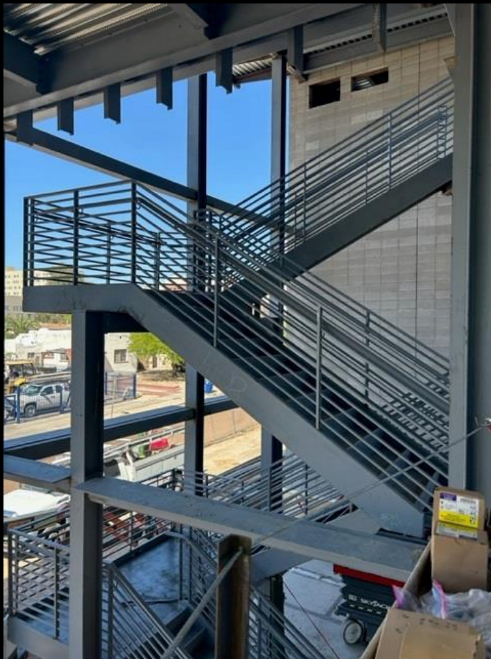
Office Building: Stairwell installed
