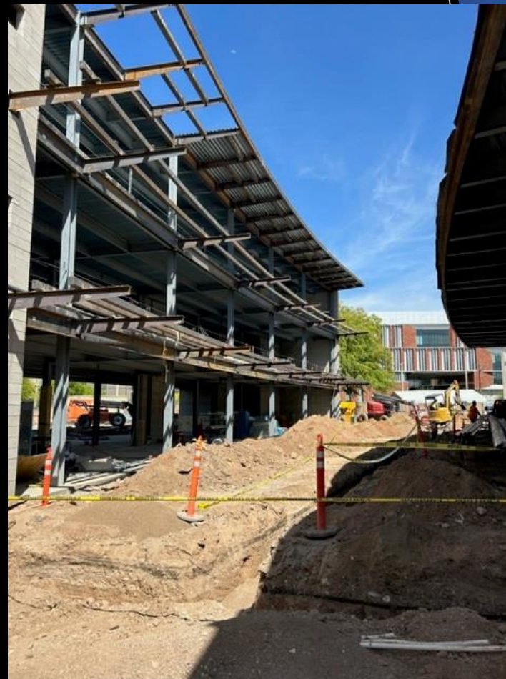
Site utilities started
