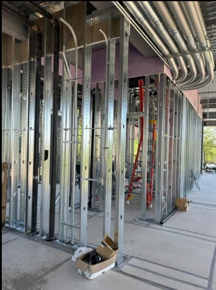
Office Building Area A: Interior framing complete and exterior framing ongoing
