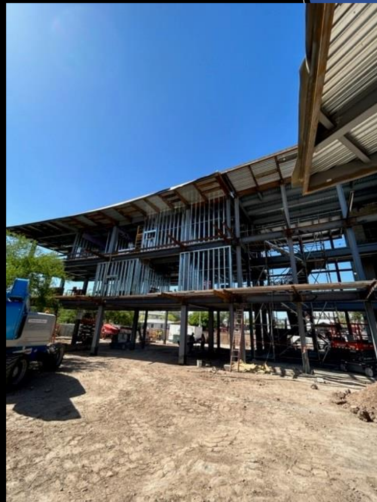
Office Building Area A: Interior framing complete and exterior framing ongoing
