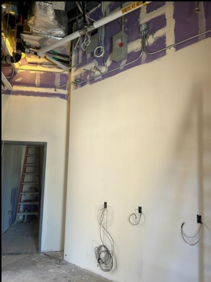
MPR building: Drywall and taping completed
