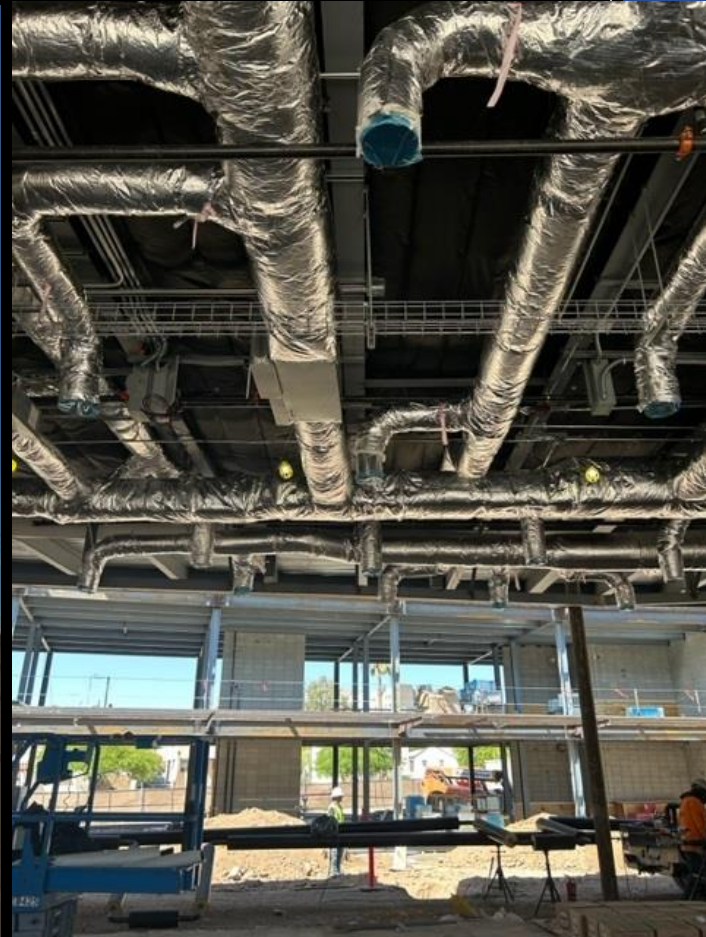
MPR building: Ductwork and deck insulation ongoing
