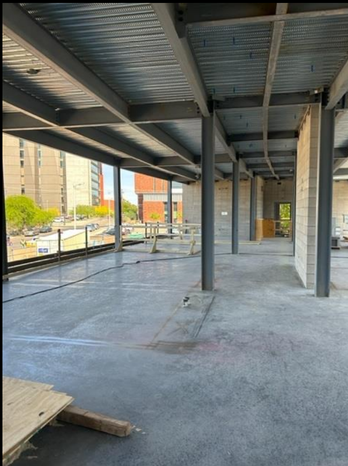
Office Building Area B&C: Level 2 & 3 Decks Poured
