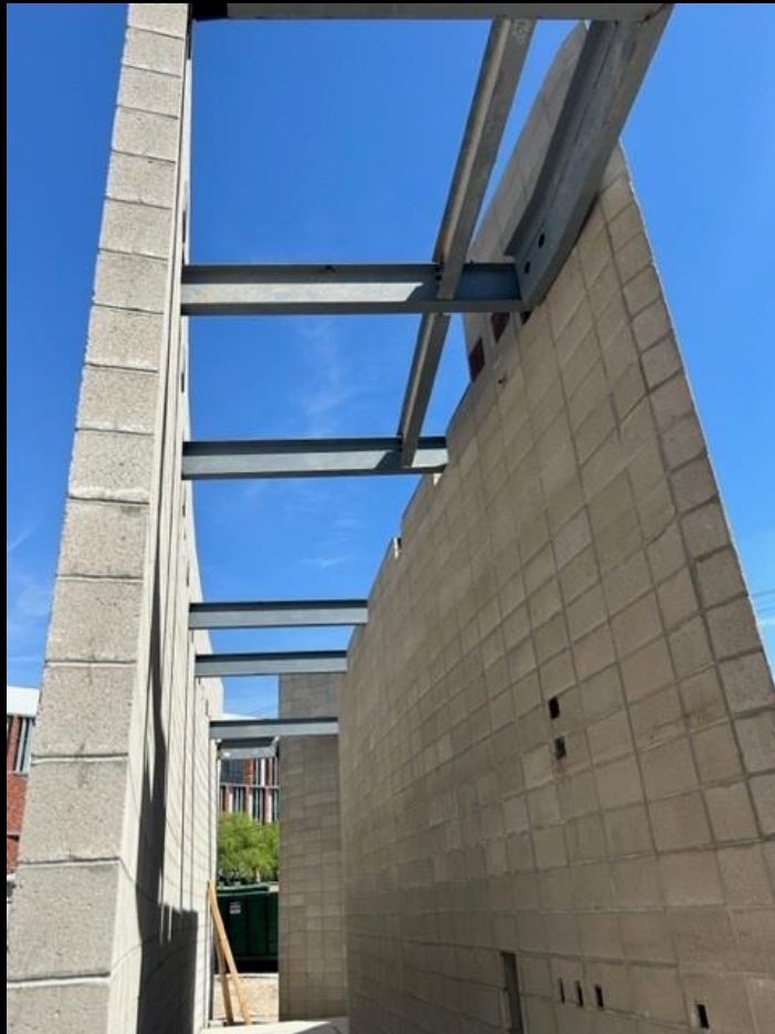
Meditation building: Steel erection ongoing
