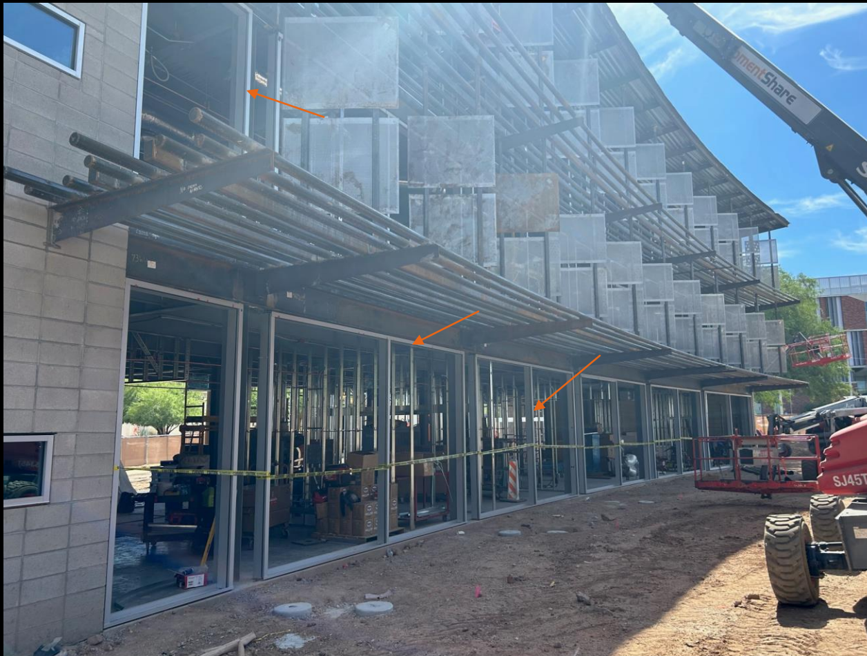
Window frames being installed in Office building
