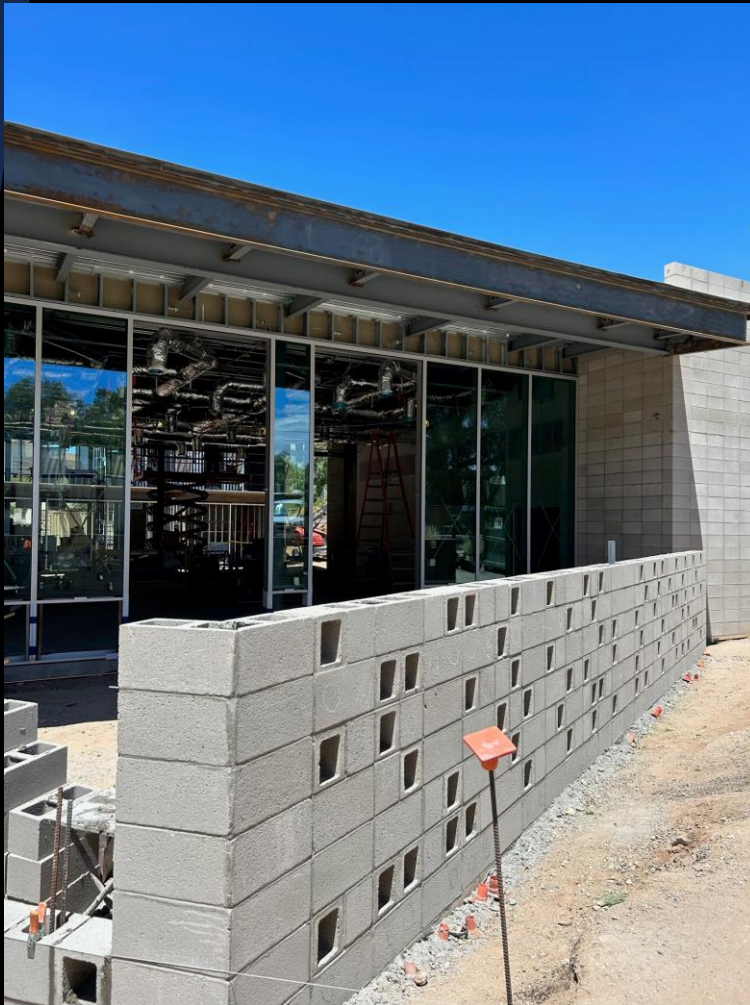
Left: Masonry screen wall ongoing in Multi-Purpose building Right: Tile finished at Multi-Purpose building
