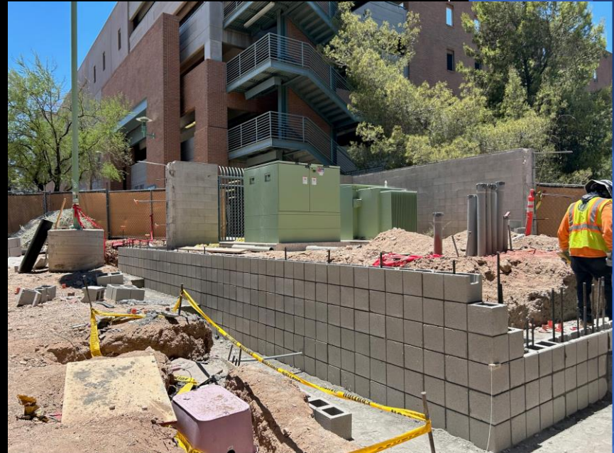
Electrical yard foundation and masonry in progress next to the Highland Garage.
