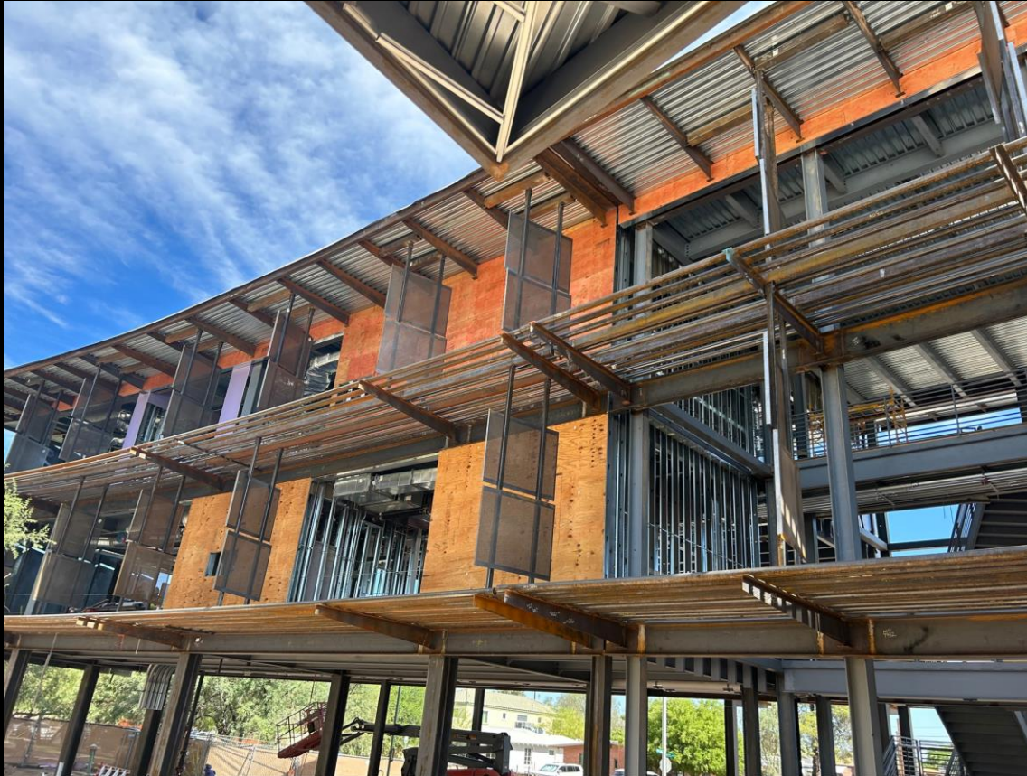
Plywood for exterior insulation finish system installed on Office building
