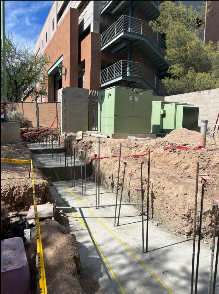
Electrical yard foundation and masonry in progress next to the Highland Garage.
