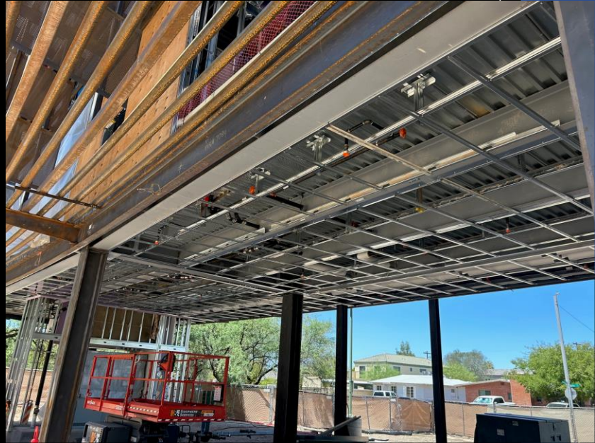
Office building: Soffit framing completed
