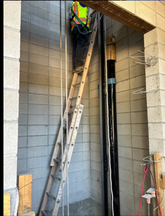
Office Bldg: Elevator rails being installed.
