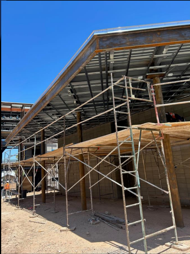
Multi Purpose bldg: Soffit framing completed, and scaffold is erected for soffit finish system.
