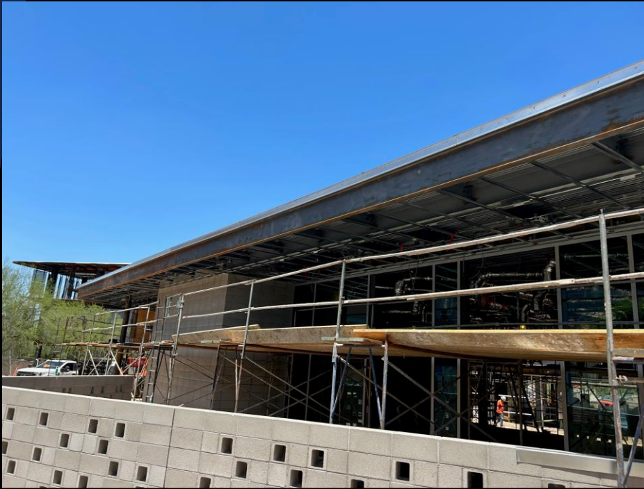
Multi-Purpose Bldg: Drip edge cleat being installed.
