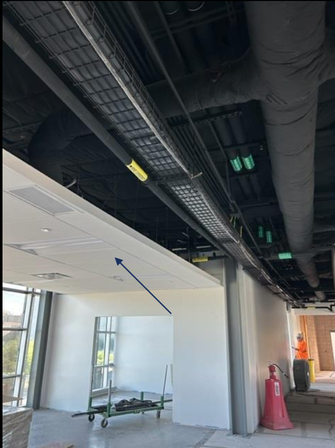
Office Bldg: Level 3 - ACT Tile installed & walls painted
