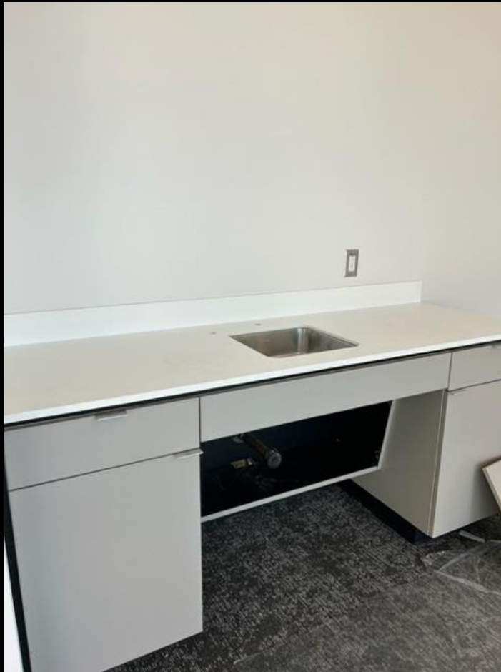
Office Bldg: Plastic laminate millwork installed
