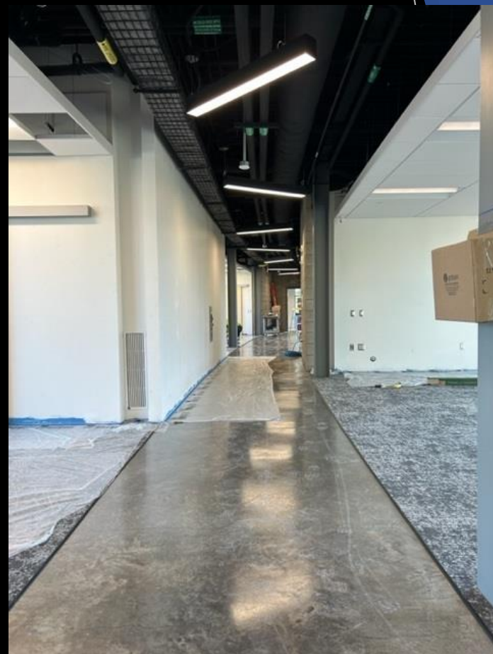
Office Bldg - Concrete being sealed in all levels. Protection installed to finishes
