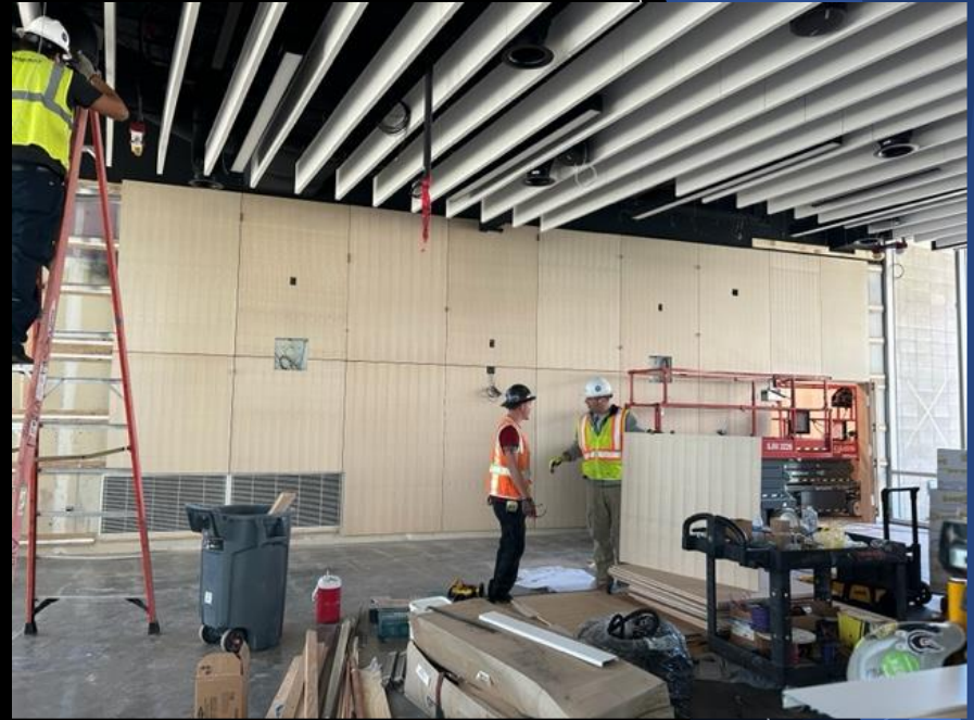
Multi-Purpose Room: Wood panels installation on-going
