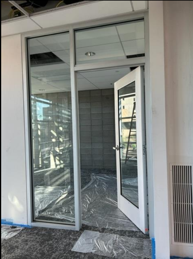
Office Bldg: Interior storefront and doors being installed in all levels
