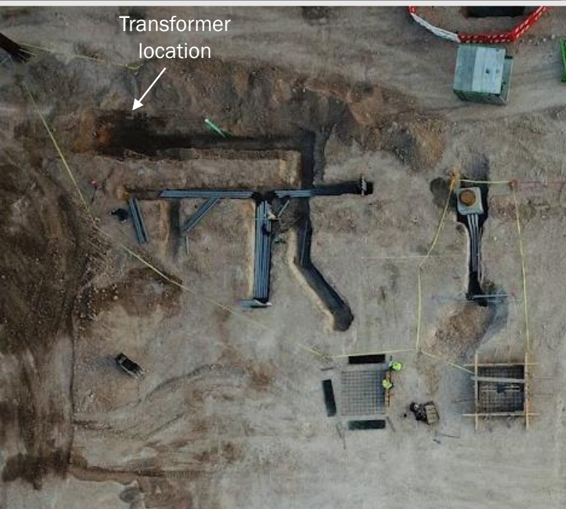
Overview of primary electrical service entering the building
