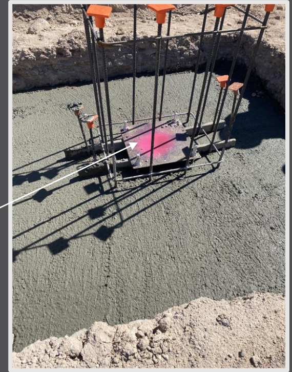
Foundation after concrete placement
