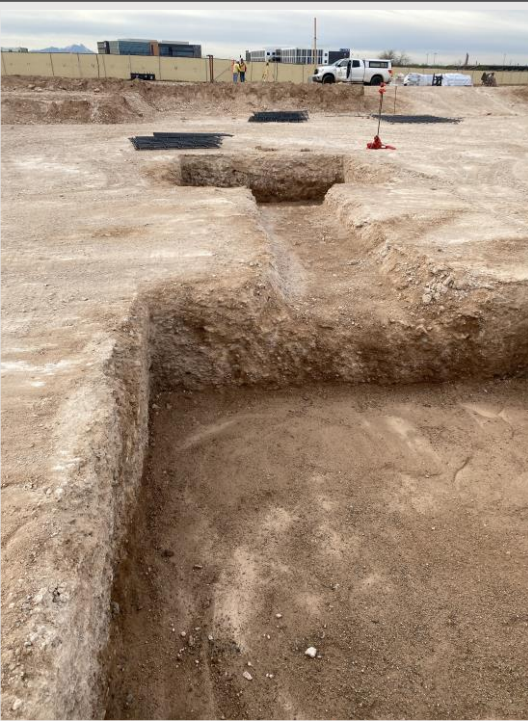
Dug foundation before rebar
