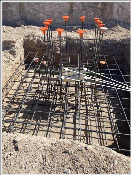
Foundation just before concrete
