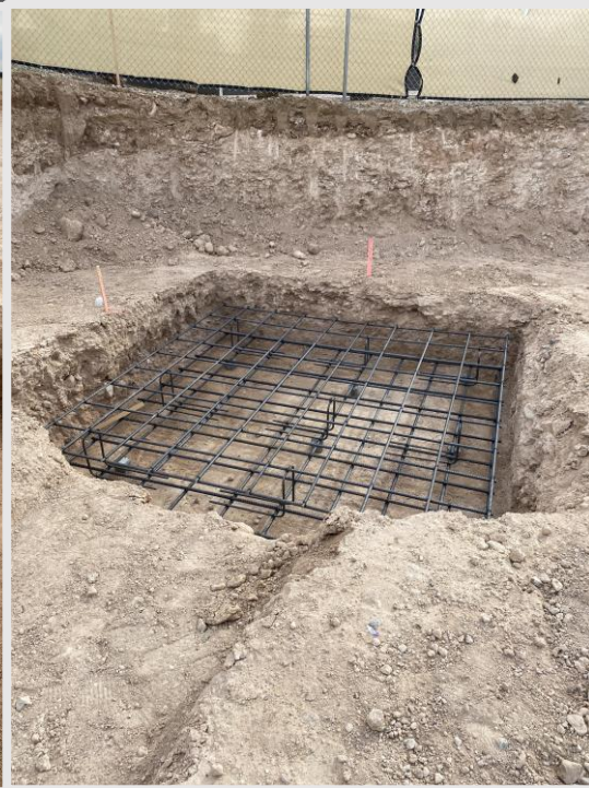
Dug foundation with 2 rebar mats
