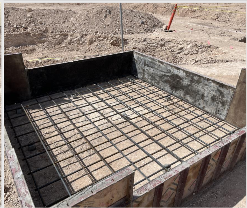
Formed foundation with single rebar mat
